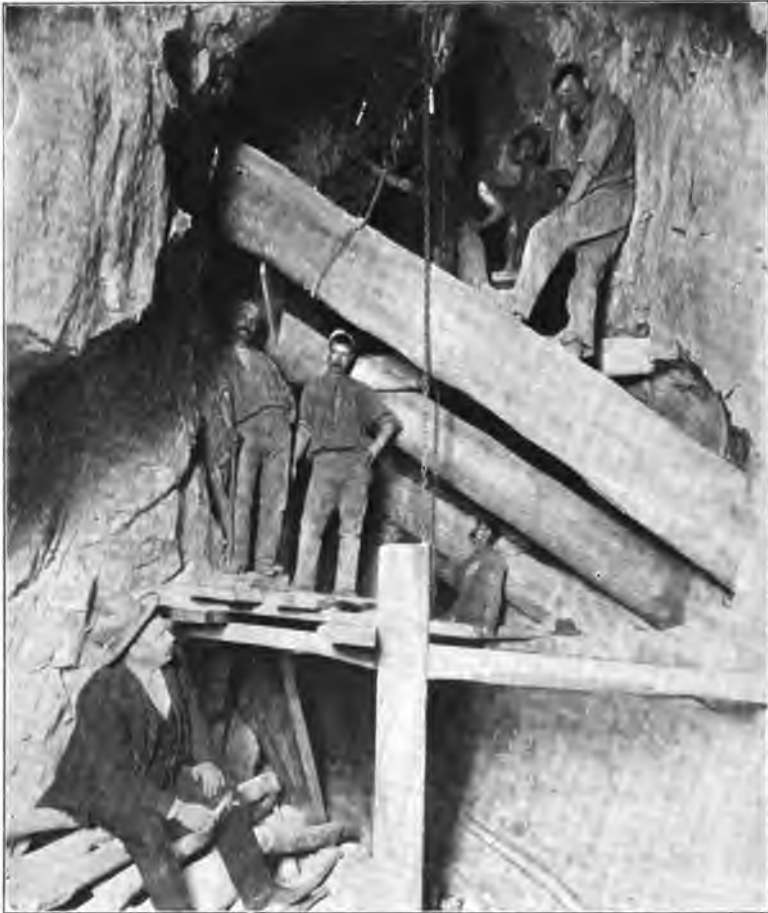
FIG. 36.—“STULL”-TIMBERING, LAKE VIEW CONSOLS.
