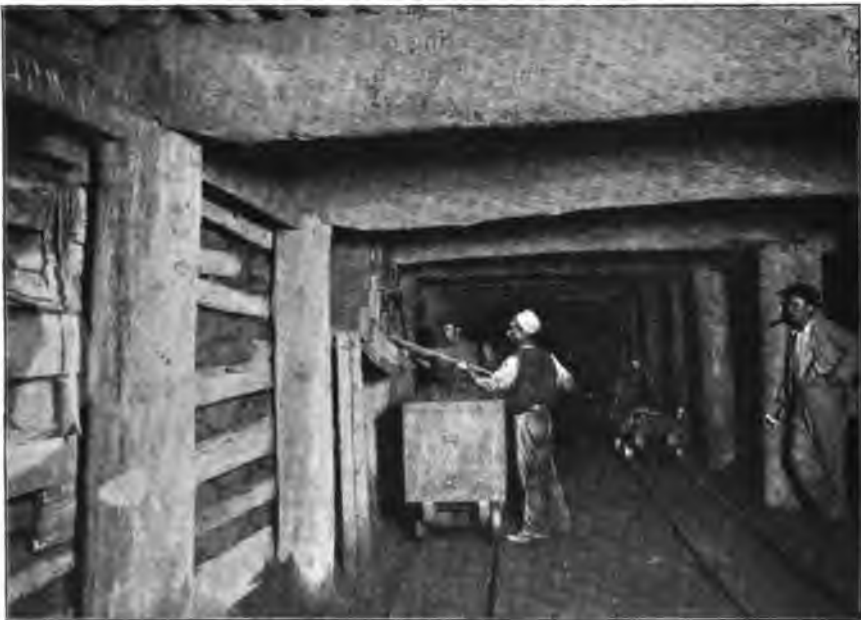
FIG. 38.—SOUTH DRIVE NO. 2 LEVEL, NO. 4 LOPE (SHOWING TIMBERING), GOLDEN HORSE-SHOE.
