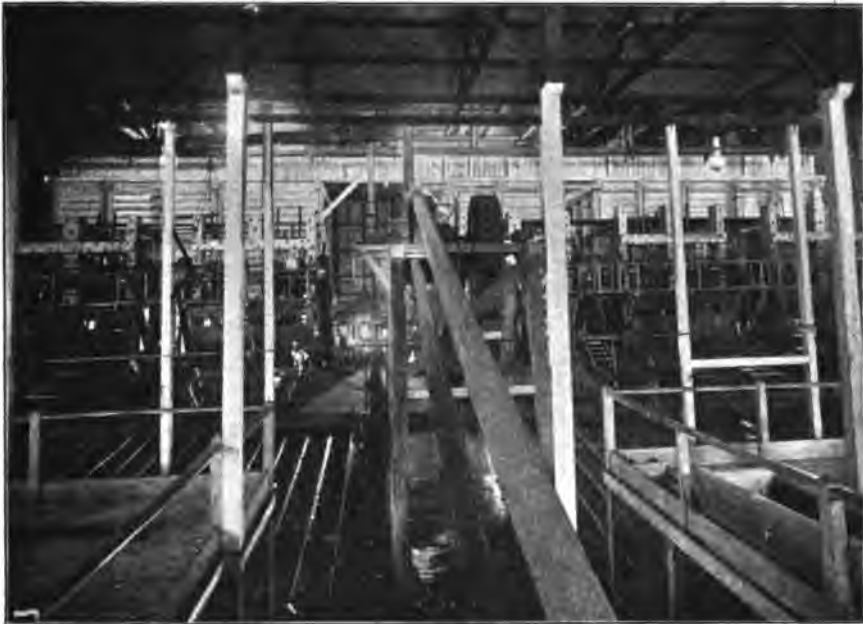
FIG. 46.—THE GOLDEN HORSE-SHOE 50-STAMP BATTERY (INTERIOR).
