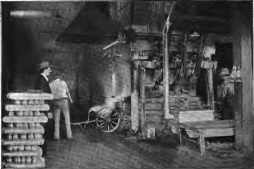
FIG. 65.—WATER JACKET FURNACE, GOLDEN HORSE-SHOE WORKS.
