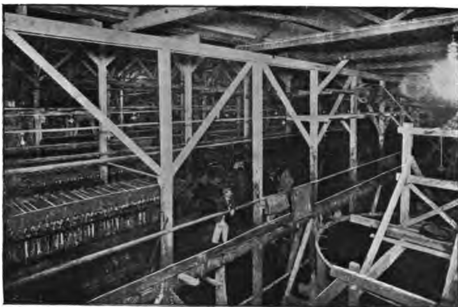
FIG. 60.—THE GREAT BOULDER CYANIDE PLANT (INTERIOR), FILTER-PRESSES AND AGITATORS.
