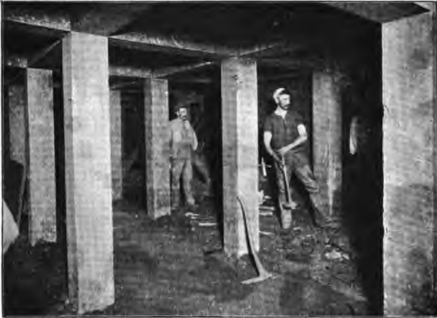
FIG. 40.—SILL-FLOOR No. 2 LEVEL No. 4 LODE (SHOWING SQUAKE-SET TIMBERING), GOLDEN HORSE-SHOE.
