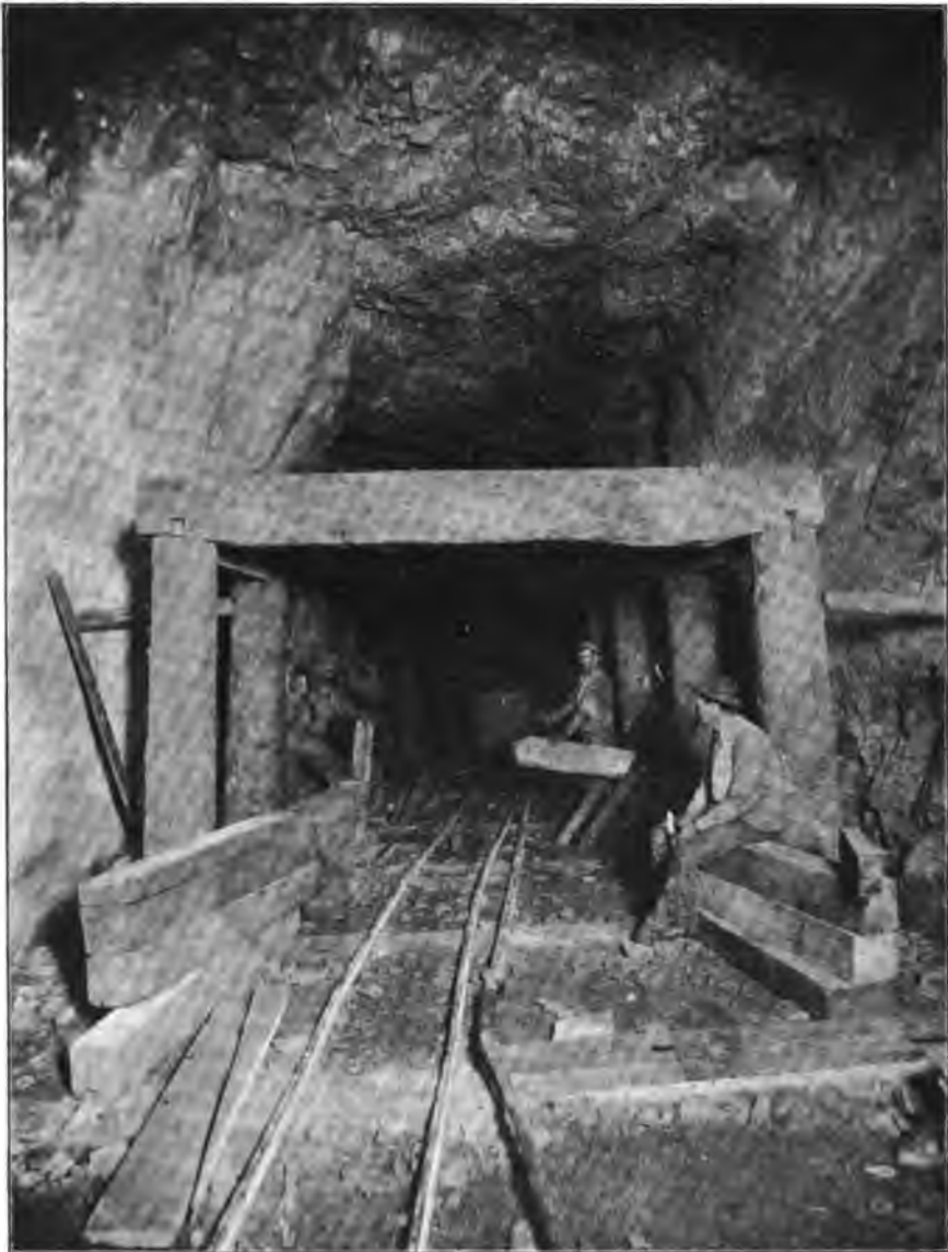
FIG. 35.—SOUTH DRIVE, 350-FEET LEVEL, SOUTH NO. 4 LODGE (LOOKING NORTH), GOLDEN HORSE-SHOE.
