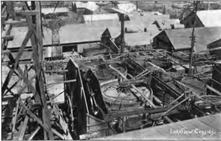
FIG. 52.—THE LAKE VIEW CONSOLS CYANIDE PLANT (SHOWING VATS WITH BUTTERS AND MEIN'S DISTRIBUTORS).
