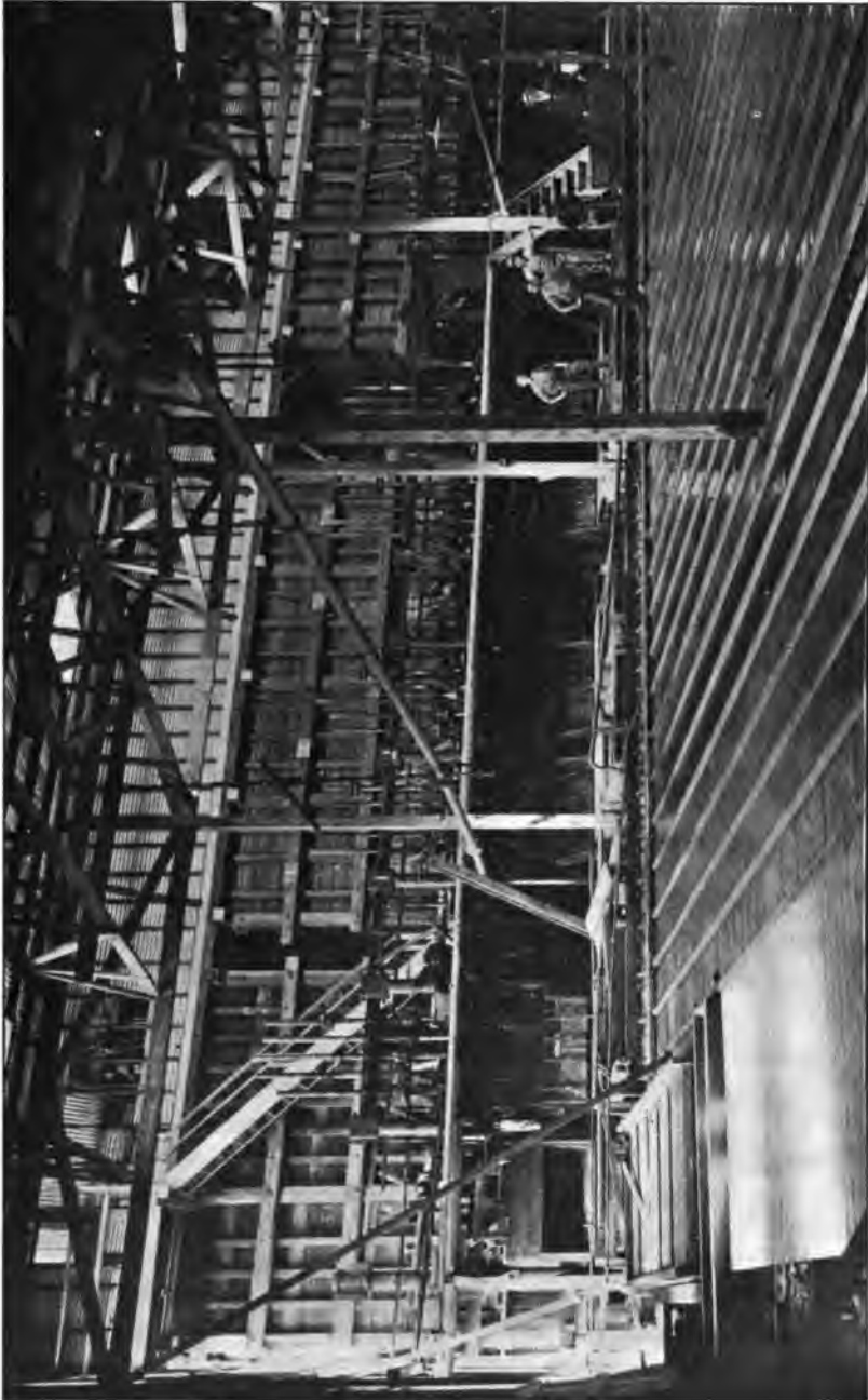
FIG. 45.—THE IVANHOE STAMP BATTERY (INTERIOR).
