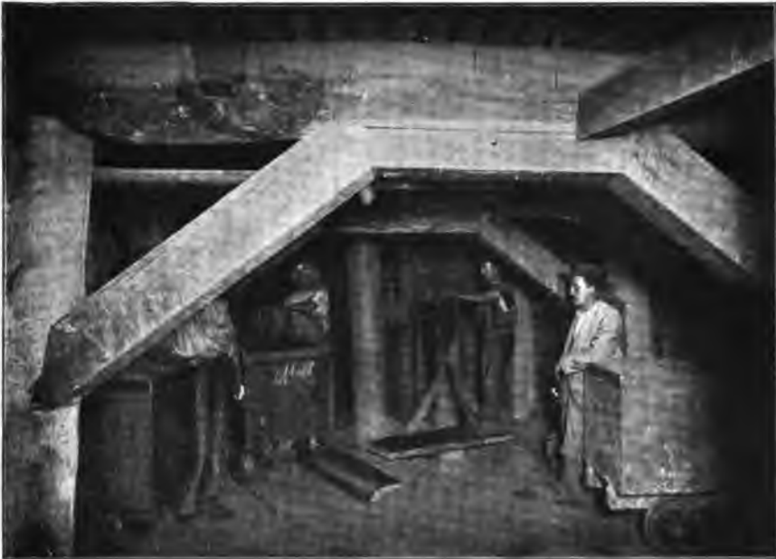
FIG. 39.—JUNCTION OF CROSS-CUT AND NO. 3 LODGE NO 1 LEVEL, GOLDEN HORSE-SHOE.
